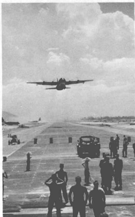
93. Runway Resurfacing—Phu Bai. Seabees of NMCB-133 resurface the runway as a C-130 Hercules aircraft takes off from the completed end of the runway.
