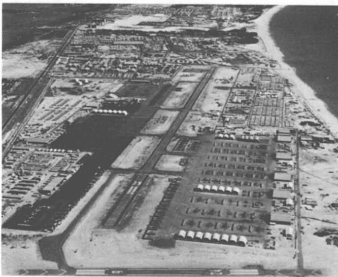
15. Marble Mountain Air Facility (MMAF)—Da Nang. This was a light plane and helicopter airfield. The original runway was 2,000 feet, built of Pierced Steel Plank (PSP). The PSP was subsequently replaced with an asphaltic-concrete wearing surface. The parking aprons were of PSP and measured 135,000 and 45,000 SY each.
