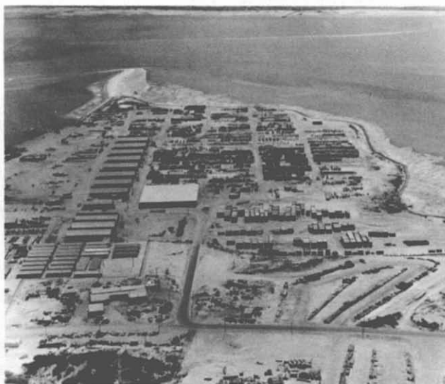
42. Cam Ranh Depot (RMK-BRJ). This major RMK-BRJ depot was begun in November 1965 with the filling of a spit in Cam Ranh Bay. The waterfront location was chosen so that LSTs and barges could be handled directly. To provide needed additional open storage space, a sand dune east of the spit was levelled and spread out to enlarge the north side of the open storage area.
