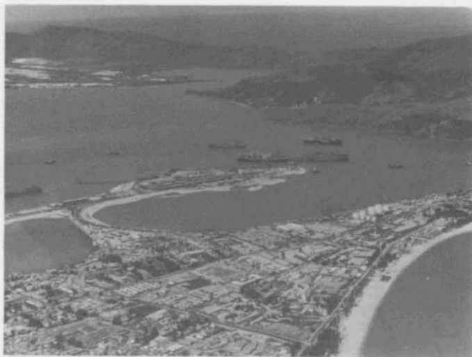
4. Qui Nhon Harbor. The man-made deep-draft facility at center of photo called for dredging an entrance channel and turning basin and depositing the fill on a Japanese constructed rock breakwater. The fill formed a 30-acre staging area. The T-shaped pier is composed of four joined mobile DeLong units.
