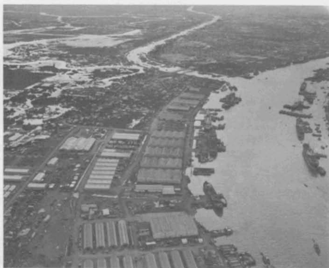
3. Saigon River Port. Note wharf "Quay 1" in the center of the photo. This 90' \times 510' structure, built by RMK-BRJ, was operational on 1 October 1966.
