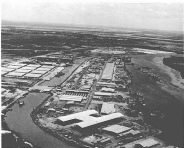
41. Saigon Island Depot (RMK-BRJ). This is Thu Duc Island—one of RMK-BRJ's 3 such depots in South Vietnam. Originally marsh land, this GVN-owned island required filling and stabilizing of 590,000 SY of area, and the hauling of 1,200,000 CY of sub-base material, and 240,000 CY of rock for surfacing the area. The Thu Duc Depot included major repair shops, warehouses, open storage areas, and marine construction facilities.
