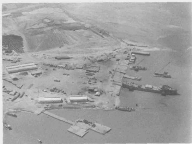
5. Tan My Port Facility. This project included 4 LST ramps, 2 LCU ramps, a barge pier, and a 160,000 SY hardstand.
