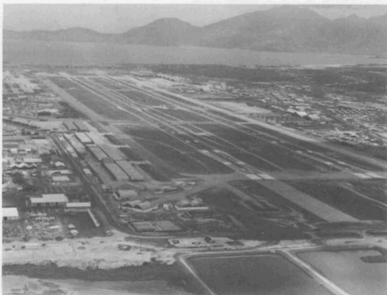
10. Da Nang Airfield. Located southwest of Da Nang, the second largest city in South Vietnam. An existing French-built 7,900' runway was modernized and re-constructed into a 10,000' jet-capable airstrip. A new 10,000' asphaltic-concrete runway was added, with 1,000' concrete touchdown sections at either end, 1,000' overruns, taxiways, and warm-up aprons. Other major items were an 80,000 SY aircraft parking apron, a 48,000 SY helicopter parking apron, and ancillary maintenance and support facilities.
