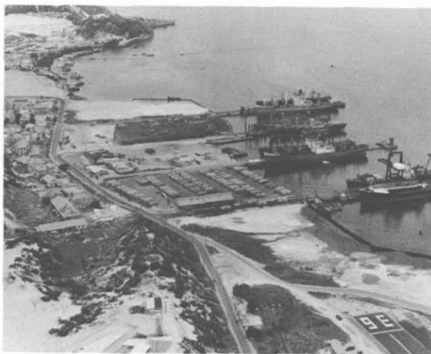
24. Cam Ranh Bay Port Facility. A deep-draft pier of steel-pile construction, 400' long by 45' wide, was built in 1963 by RMK. Between 1965 and 1967, the Cam Ranh Port evolved into the extensive facility shown in the photo. By May 1967, the Port could handle, simultaneously, 8 deep-draft cargo vessels, plus one POL tanker. Army troop units installed the sheet-pile bulkheads and stabilized the contractor-dredged fill for use as staging areas. Three of the piers are of the DeLong type.
