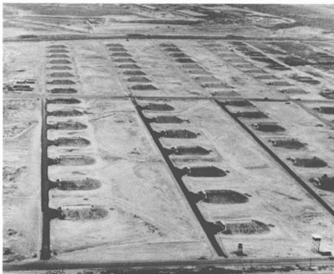
31. Ammo Storage Facility at Long Binh. These massive earth-covered concrete and steel Stradley ammunition bunkers were among the final projects completed by RMK-BRJ.
