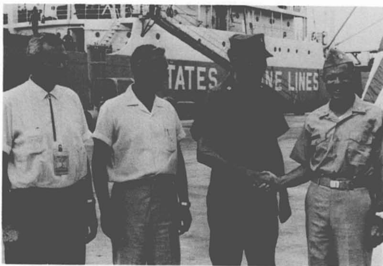
61. Newport Project Key Personnel. Four key members of the military-civilian construction team responsible for "Newport" were: (for RMK-BRJ) James A. Lilly, General Manager; Bert L. Perkins, Operating Committee Deputy Chairman; (for NAVFAC) LT Paul McCullagh, Resident Officer-in-Charge of Construction; and RADM Spencer R. Smith, Officer-in-Charge of Construction for the Naval Facilities Engineering Command.
