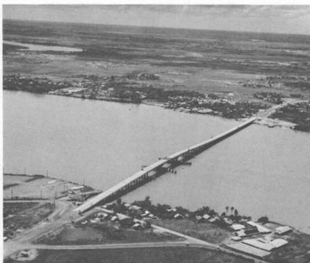
53. Bien Hoa Bridge. This is the largest of the 6 bridges which comprised a major bridge building program ($20 million) in the Saigon area. The Bien Hoa span is 2,631 feet long; it crosses the Dong Nai River on QL 1, 17 miles northeast of Saigon. It was started on 15 May 1971 and was completed on 1 May 1972, at a cost of $4.5 million.
