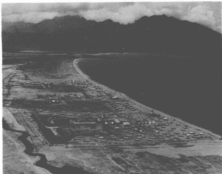
80. Camp Haskins—Da Nang. Aerial view of Camp Haskins, Red Beach, Da Nang, looking north, showing NMCB-1 cantonment, the 30th NCR Headquarters, and NMCB-9 camp in the background.
