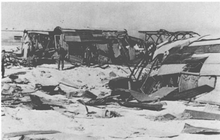
85. Viet Cong Attack on Hospital—Da Nang. View of destruction of a segment of the new U.S. Naval Hospital, Da Nang—then under construction by NMCB-9. The hospital, and an adjacent Seabee camp, were attacked by the Viet Cong on October 28, 1965. During the attack, two men were killed and 93 were wounded. The Seabee camp was subsequently named "Camp Adenir"—in honor of SD3 Restituto P. Adenir, who was killed in that attack.
