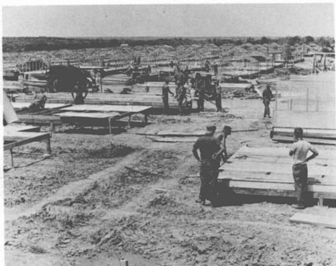
72. "Strongback Huts"—Quang Tri Combat Base. Seabees of NMCB-11 are building hundreds of "Strongback Huts" for a Marine camp. These units were later converted to "SAE Huts" by replacing the tenting with corrugated sheet metal roofing.
