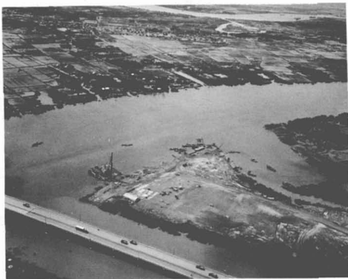
17. Newport (Saigon)—Early View. A rice paddy, two miles north of Saigon, was selected for a "new port" to alleviate the jam-up of freighters waiting to unload—some, as long as 30-40 days. The pile driver barge in the photo is in the process of driving 1,144 piles to form the shallow-draft section of the port. Some 500 of these piles had to be driven an average of 135 feet.
