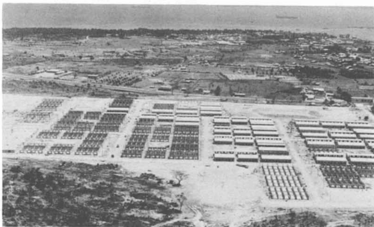
28. USAID Housing at Cam Ranh Complex. Construction of Community Housing at Cam Ranh Bay for Vietnamese tenants. Included in the Project were an Administrative Building, Fire Station, Elementary School, and Market Building; also, sewage collection and treatment, water supply and distribution, and power distribution.
