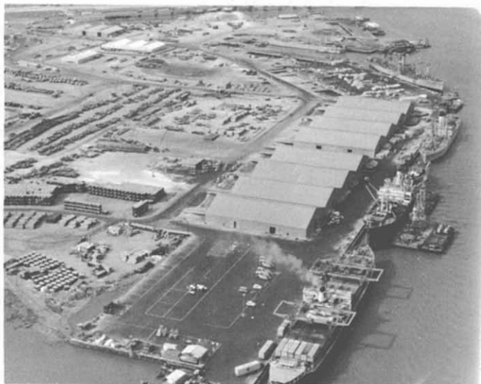
20. Newport (Saigon)—Close-up View. This is the deep-draft concrete wharf. The 4 berths have a combined length of 2,400 feet; the 8 transit sheds have a total floor space of 192,000 SF.
