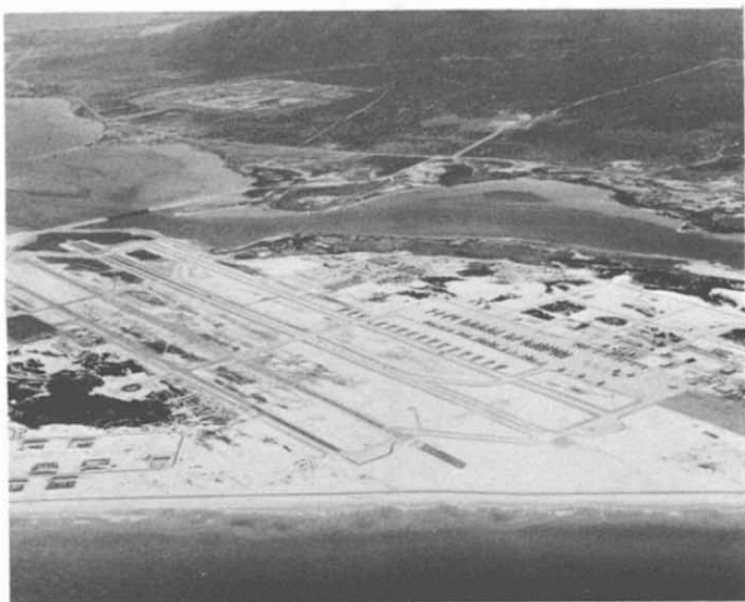
22. Cam Ranh Airfield—Completed. The 17-mile Cam Ranh Peninsula is characterized by rolling sand dunes. The original 10,000' interim (expeditionary) runway/taxiway was constructed of AM-2 (aluminum matting), shown in the left half of the airfield in the photo. A parallel permanent 10,000' concrete runway/taxiway was then added to complete the basic airfield.
