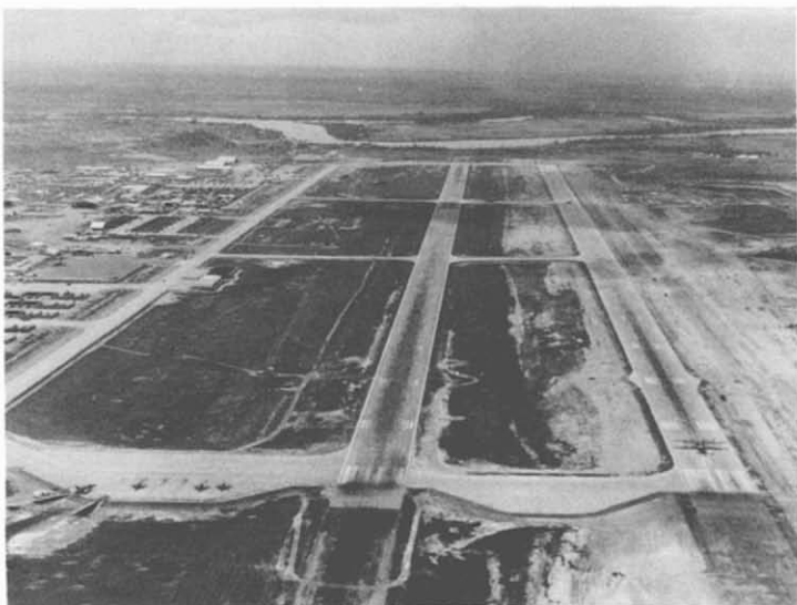
12. Bien Hoa Airfield. Located about 15 miles northeast of Saigon. Bien Hoa was the only military airfield in Vietnam prior to 1965. A 10,000' concrete runway and taxiway was built by RMK in 1963. A parallel 10,000' concrete runway was added in 1967.
